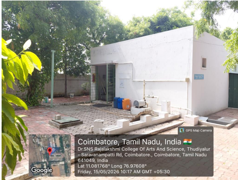
Sewage Treatment Plant (STP)
